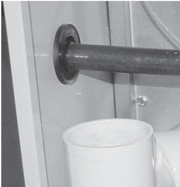
Figure 23 - Furnace Gas Pipe Connections (Note Rubber Grommet)
