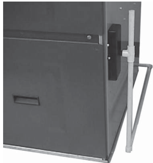
Figure 21 - Condensate Trap/Condensate Drainage With Vent
