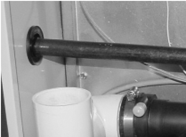
Figure 28 - Furnace Gas Pipe Connections (Note Rubber Grommet)
