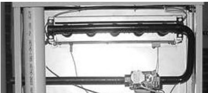
Figure 29 - Inshot Burner Assembly
