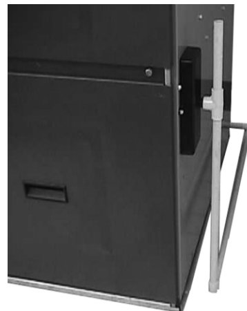
FIGURE 26 - CONDENSATE TRAP/CONDENSATE DRAINAGE WITH VENT
