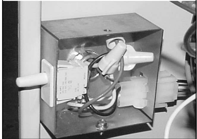
FIGURE 36 - INTEGRATED HOT SURFACE IGNITION CONTROL
