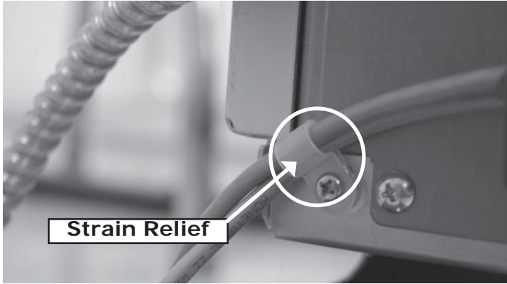
Figure 9-9 MCHP Low Voltage Wiring Strain Relief
