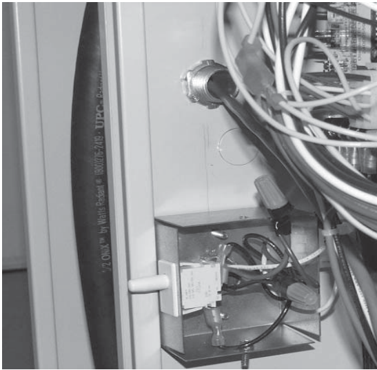
Figure 14-6 240 VAC MCHP Connections
