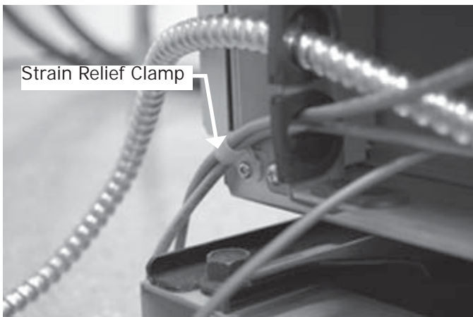
Figure 10-13 MCHP Communication Cable & Exhaust Leak Sensor Cable
