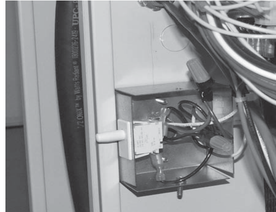
Figure 10-5 120 VAC Furnace Connections
