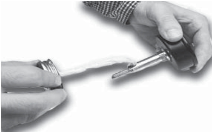
Figure 7 - Apply Pipe Sealant On Shaft of Gauge
