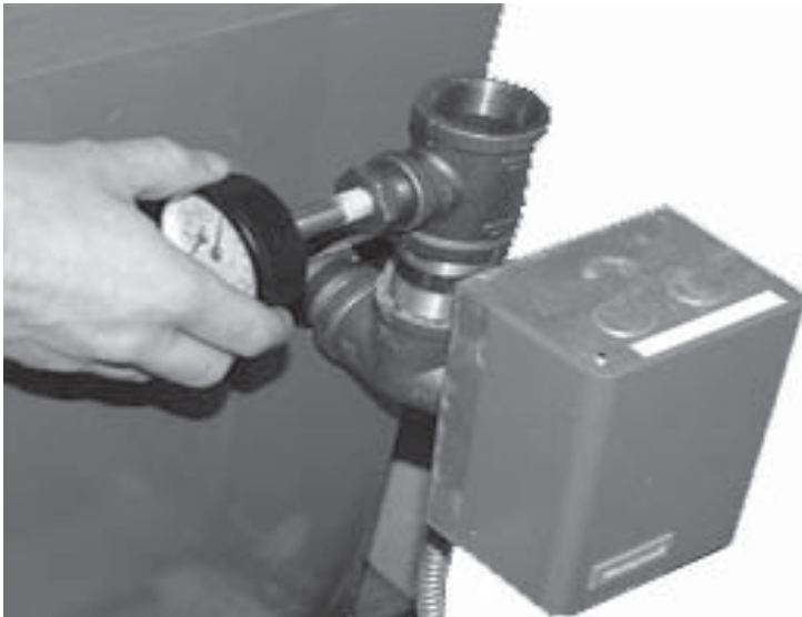
Figure 8 - Thread Gauge Into Supply Water Tee
