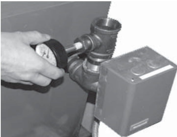
Figure 8 - Thread Gauge Into Supply Water Tee
