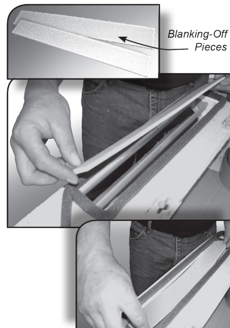
Figure 6 - Applying Blanking-Off Pieces
