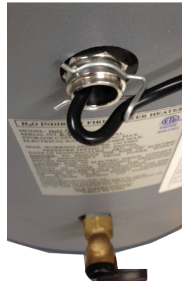
Figure 3 - Sensor Wire Secured to Well With Clip
