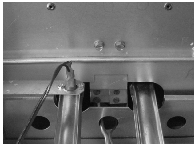
Figure 5 - Install Burner Door and Tubes (3 Section Shown)
