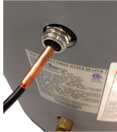
Figure 4 - Secure Sensor Wire to Well With Clip
