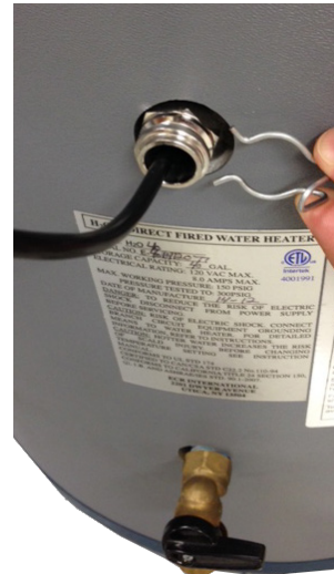
Figure 5 - Sensor Wire Secured to Well With Clip
