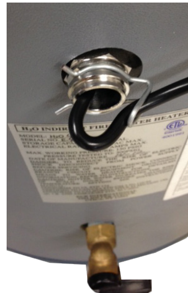
Figure 5 - Sensor Wire Secured to Well With Clip
