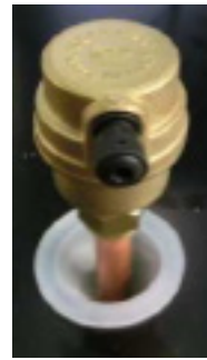
AERATOR - LOCATED ON TOP OF BOILER
