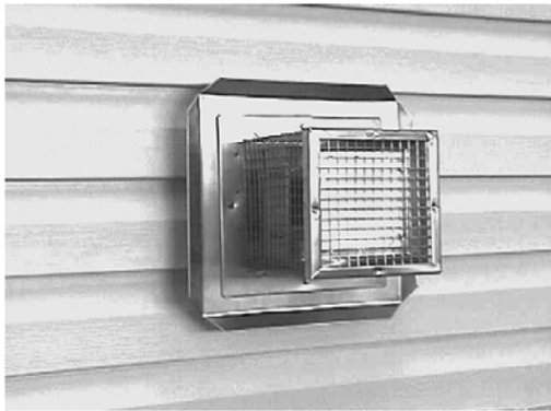
Typical Standard Vent Terminal Installation.
