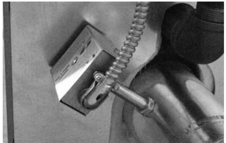
**Figure 3 Acceptable Mounting Position 2**
