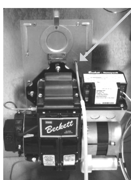
Over-fire draft access port.
