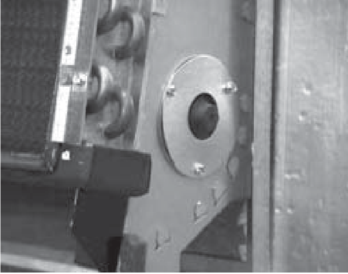
Figure 12 - Finished View Of Retainer Ring Installed Onto Bearing
