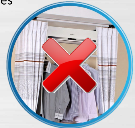
Obstacles prevent proper airflow
