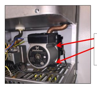
Remove 4 Allen bolts to remove motor from housing
